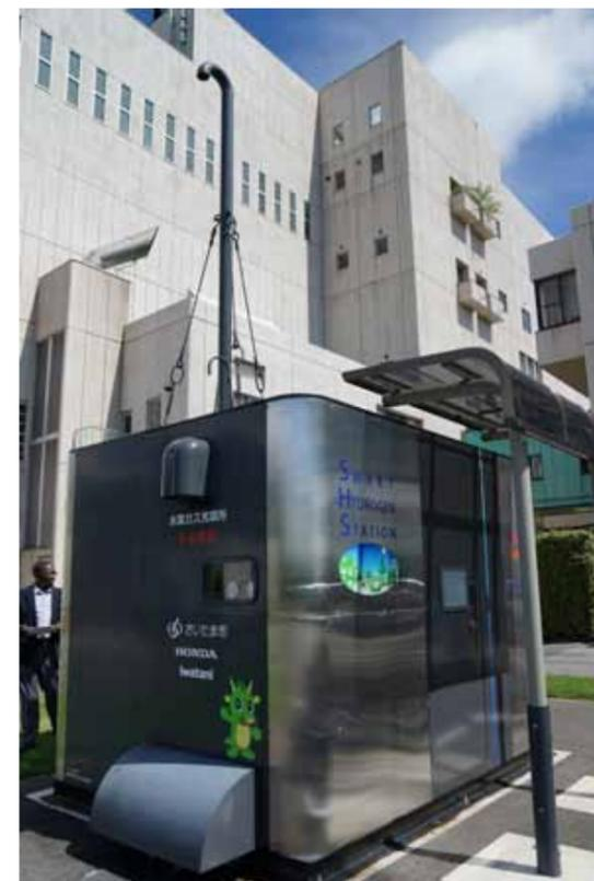
Honda's Smart Hydrogen Station (SHS) is a compact hydrogen refilling station with self-hydrogen generator from solar, biomass or other renewable energy. In a time of disaster, this SHS can provide electricity to community through the power unit in their fuel cell vehicle.
